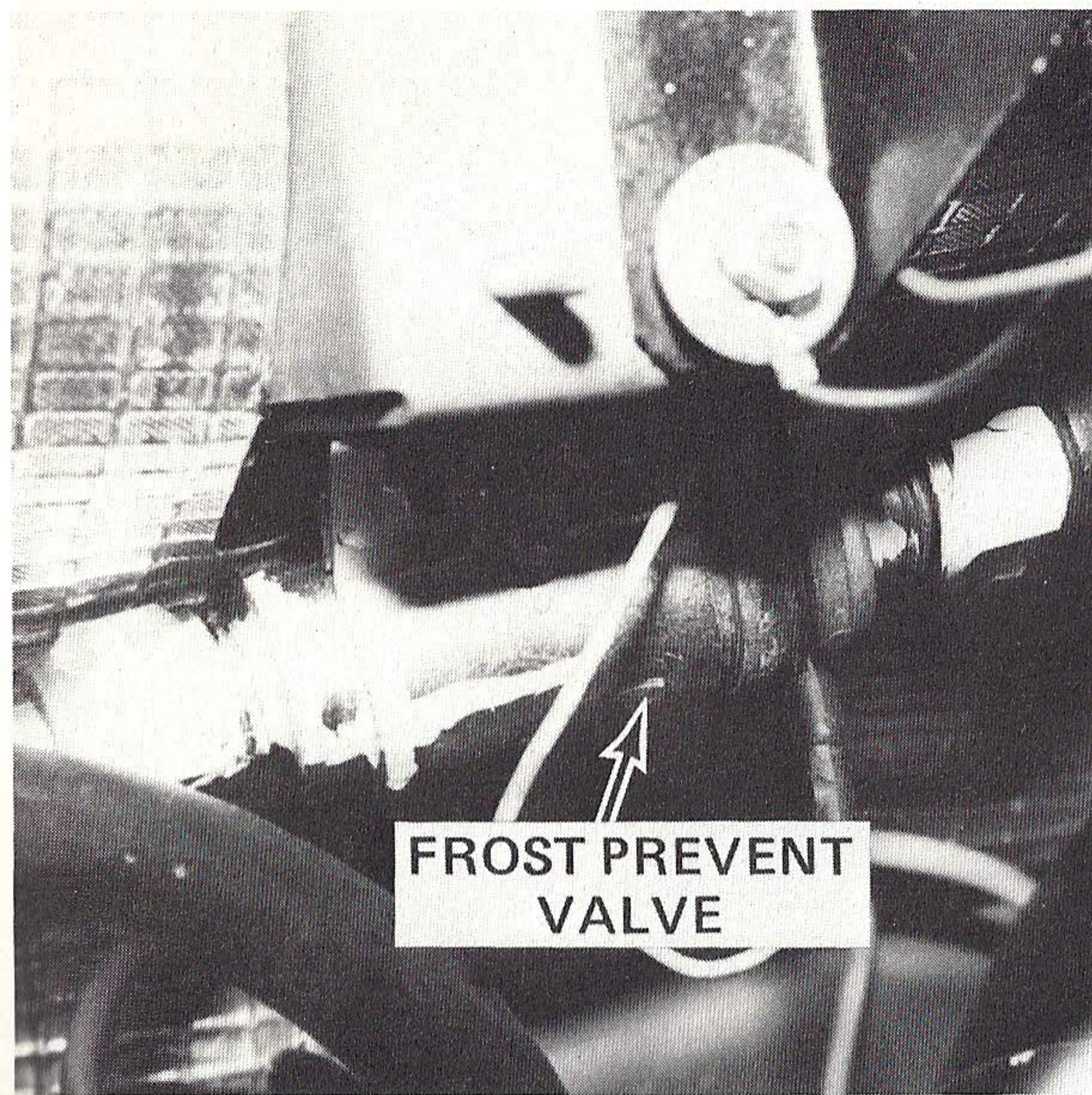
Figure 1—Front LH Engine Compartment
